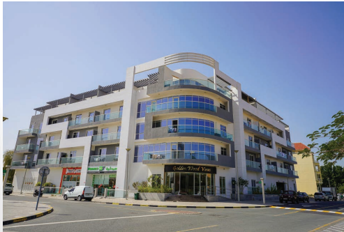
GOLDEN WOOD VIEWS JVT PROJECT LOCATION: JVT LAUNCHED 2019, COMPLETED 2020
