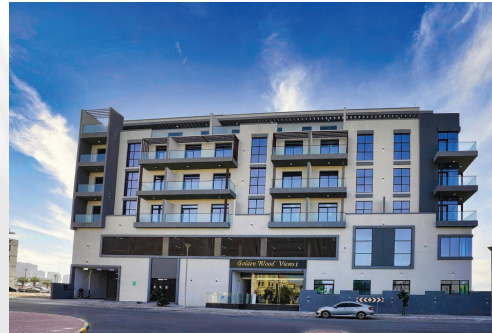
GOLDEN WOOD VIEWS 1 JVT PROJECT LOCATION: JVT LAUNCHED 2021, COMPLETED 2022
