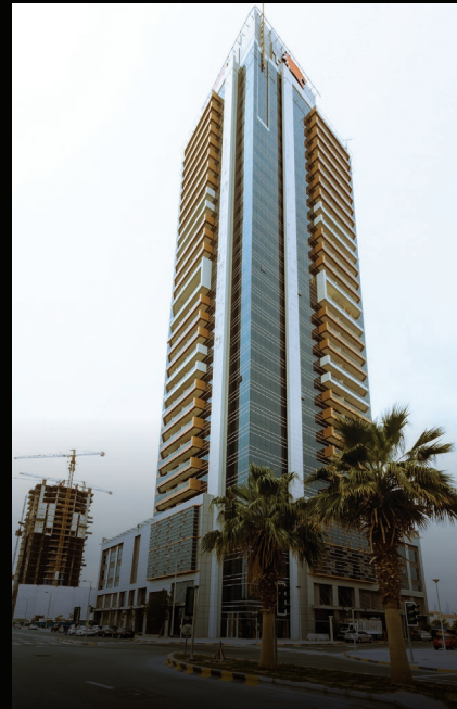
Al Manarah Tower JVT Dubai
