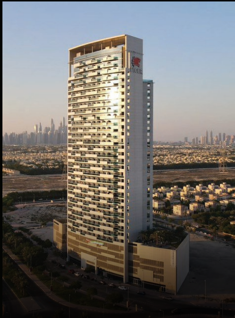
Al Jawahara Tower JVT, Dubai
