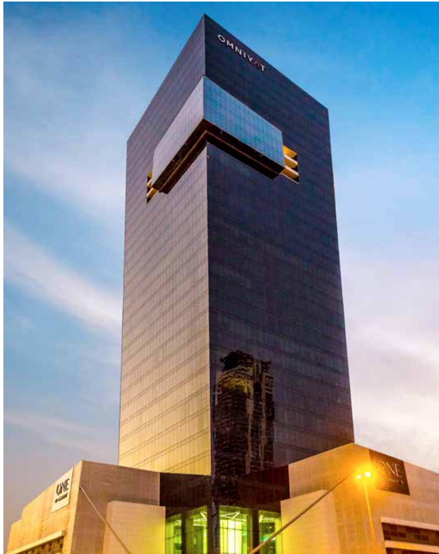
ABOVE: ONE BY OMNIYAT, OMNIYAT'S NEW SIGNATURE COMMERCIAL TOWER, LOCATED JUST OFF SHEIKH ZAYED ROAD AT THE ENTRANCE TO THE BURJ KHALIFA DISTRICT.
