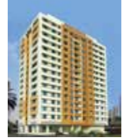
FRANKFURT SPORTS TOWER 1 HANDLED OVER
