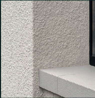
3 - PLASTER WITH PAINT
