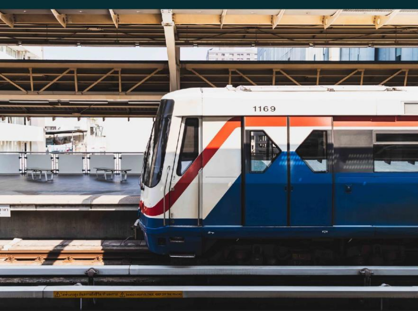
BTS SAI LUAT STATION
