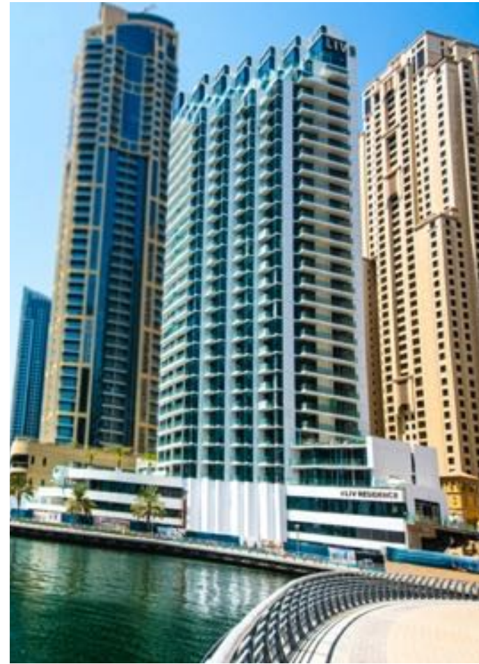
LIV Residence COMPLETED & HANDED OVER
