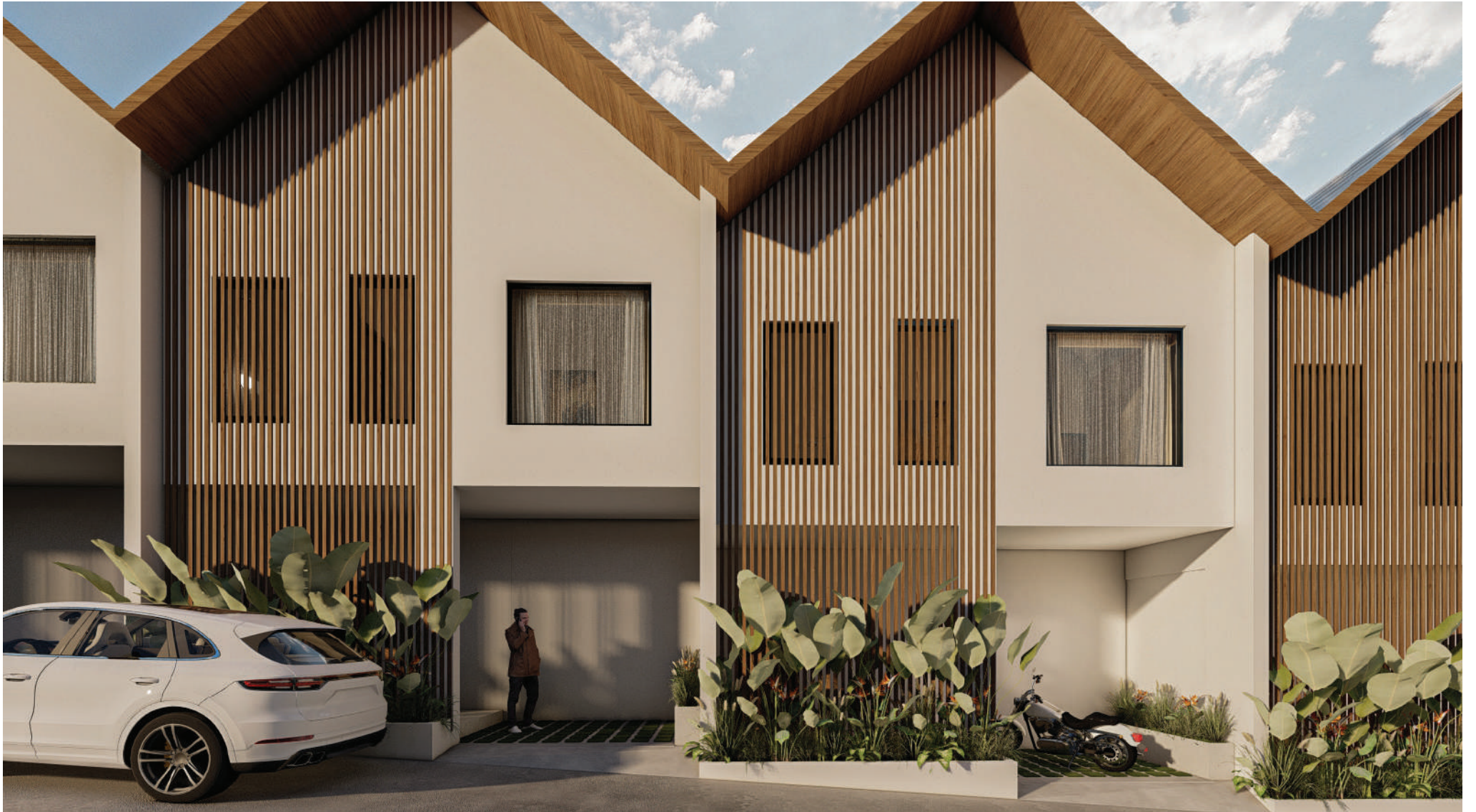
2 LEVELS ENTRANCE VIEW
