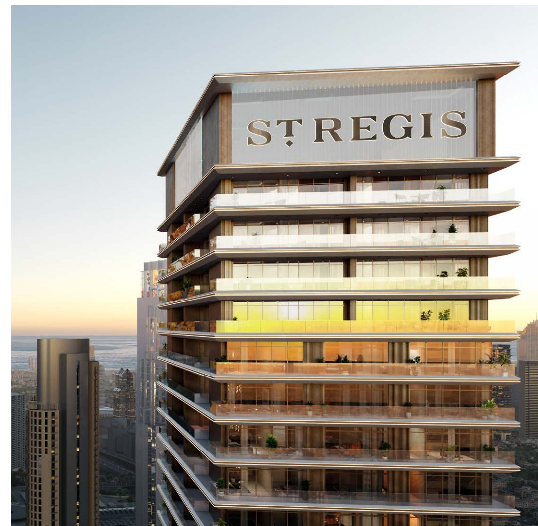
THE ST. REGIS RESIDENCES, FINANCIAL CENTER ROAD, DUBAI
