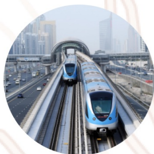
Al Jaddaf Metro Station
