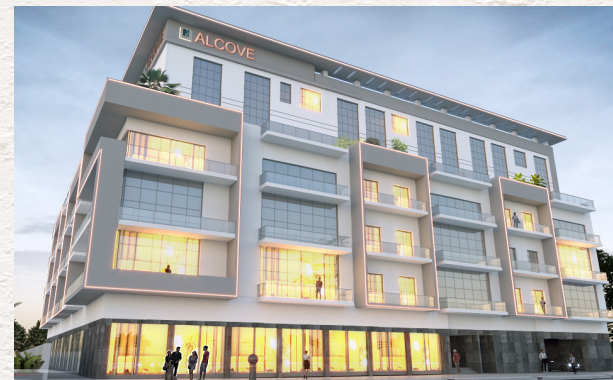
ALCOVE, JVC completed 2016 www.grovy.ae/alcove
