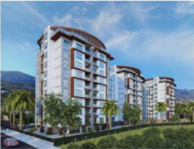
MERIT TRIO TOWERS
