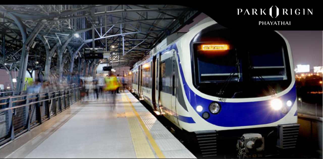
AIRPORT RAIL LINK : PHAYATHAI STATION
