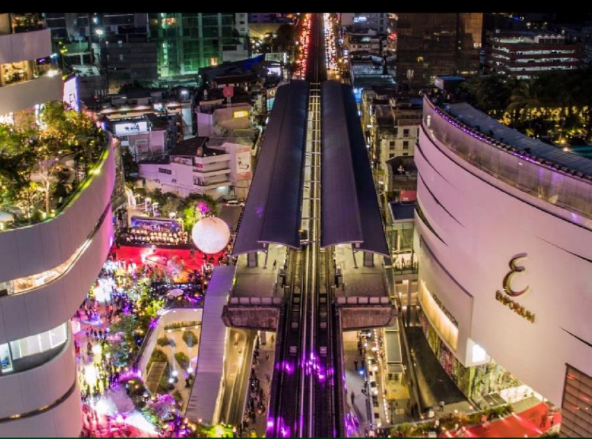
BTS PHROM PHONG STATION
